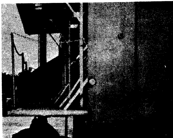
Figure 31. Chain guard railing installation.
